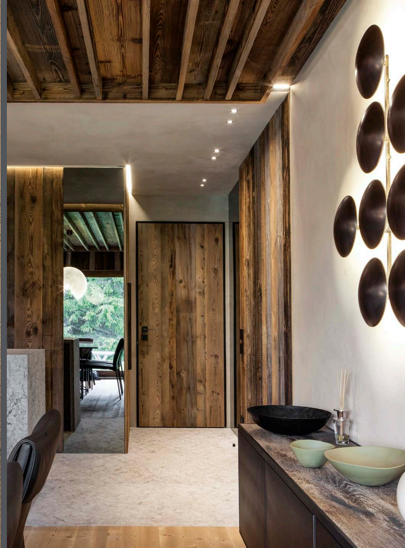
External: Customized panel with two moldings in wood according to sample Internal: Customized panel with vertical slats reclaimed wood Fitting flush with the internal wall, frame and leaf profiles and accessories with matching RAL 9005 finish
