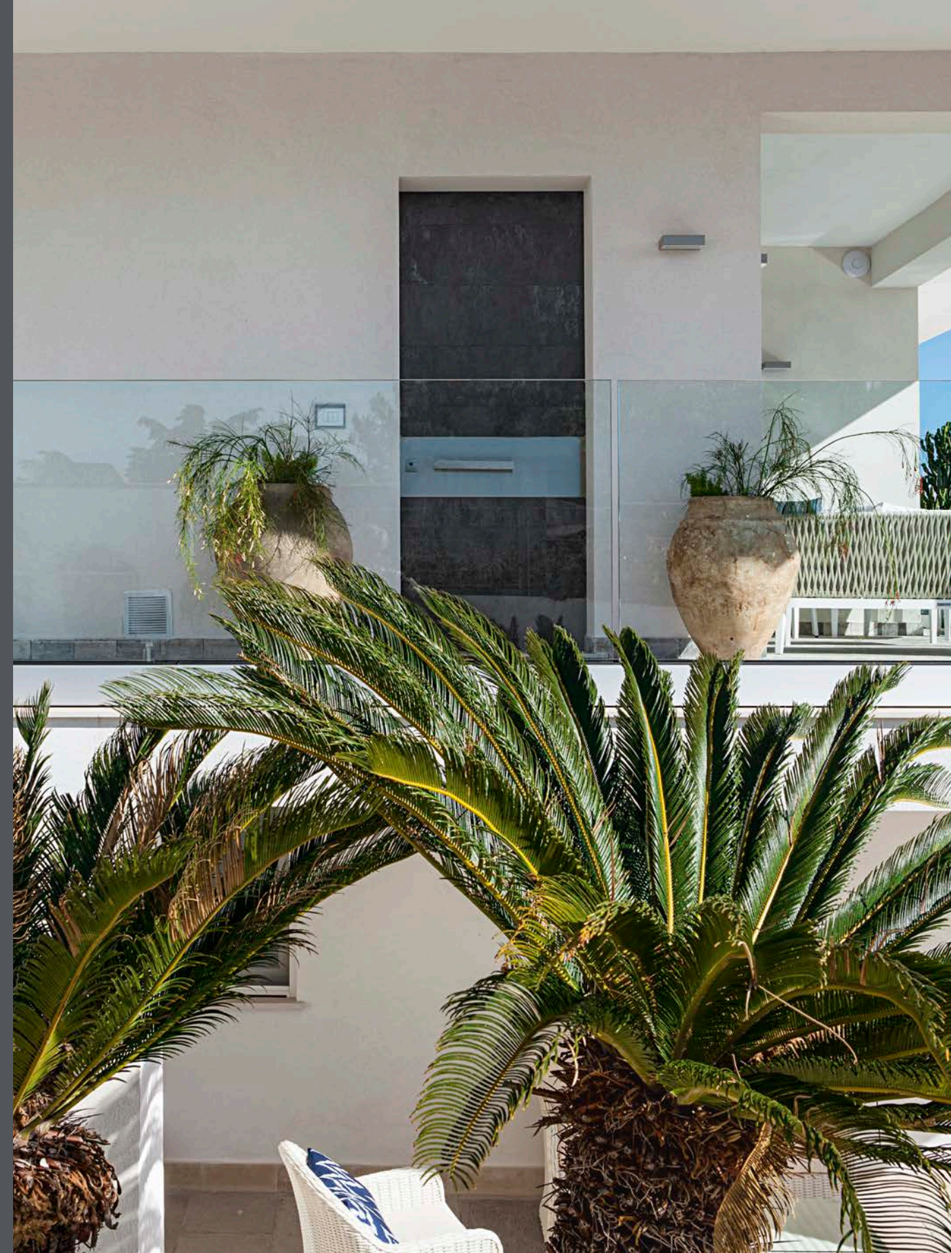
External: Tekno HTL line with Steel Laminam CorTen sectors and a stainless steel sector
