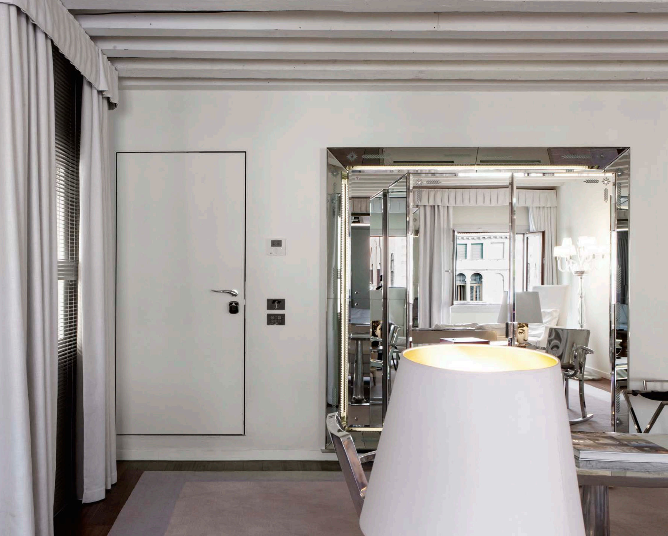
External: Piano line, polished polyester lacquered Anthracite Internal: Piano line, finished with wall painting on site Door with E130 fire-break kit and application of the Hotel locking system
