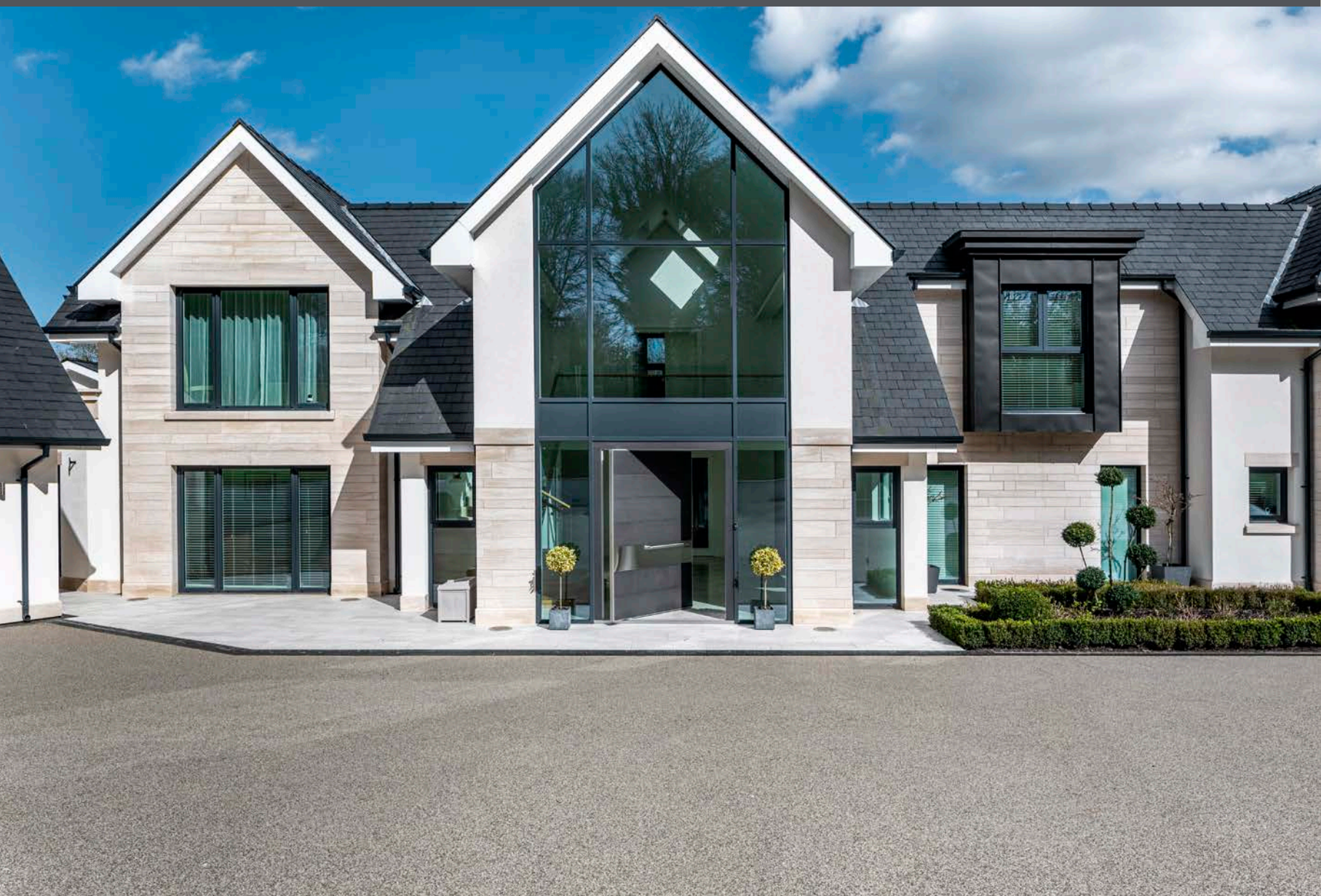
External: Portici line with open pore Oak sectors according to sample and with a stainless steel sector Internal: Portici line according to drawing, White Laminam Statuario Venato, with stainless steel sectors Fitting on the existing façade
